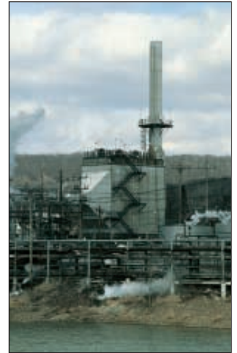
Oil refinery catalytic cracker
