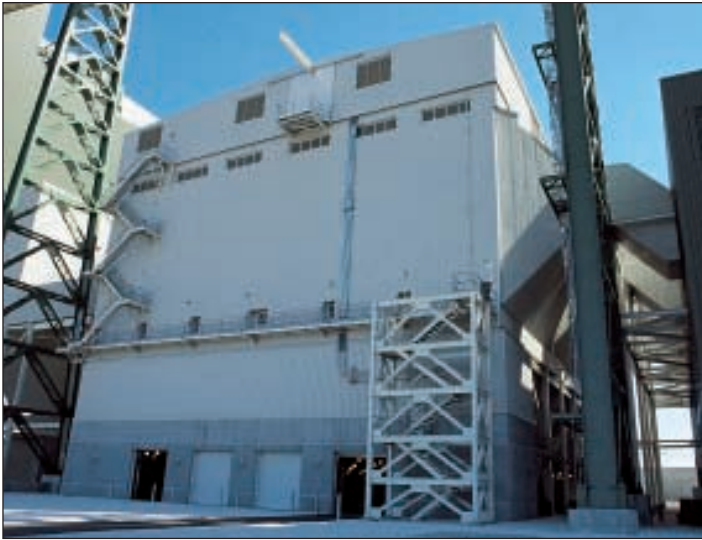
435-megawatt coal-fired power boiler
