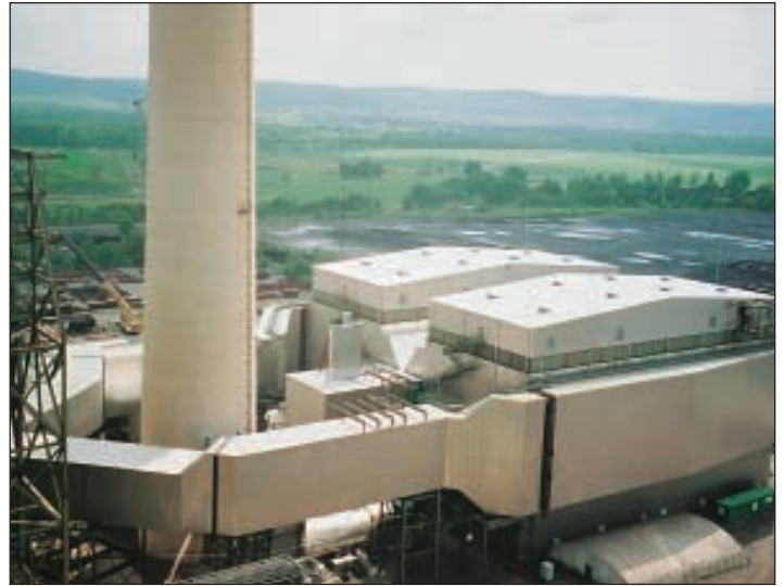
Two 745-megawatt coal-fired power boilers
