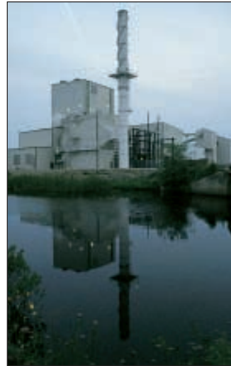
Wood-waste-fired cogeneration facility
